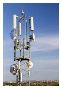
The base stations can be free standing, or mounted on top of buildings. In cities, there are often small systems mounted on the sides of buildings. The base stations have a relatively short range and so establishing a mobile phone network is a complicated and expensive undertaking, in order to ensure that population centres are covered. It is also necessary to build and operate base stations alongside motorways and other major roads.
