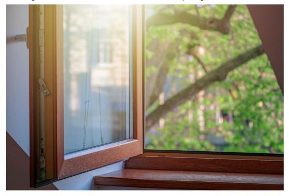
uPVC and aluminium frames are made out of preformed sections of material. These are supplied in long lengths with standard widths and heights. These sections can be cut to specific lengths to build frames to the exact dimensions required by the customer.
